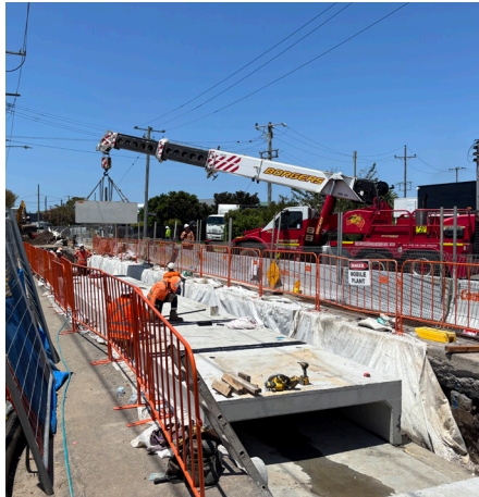
Image: culvert installation at Waratah
