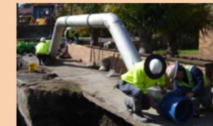
Our crews repairing a suburban water main
