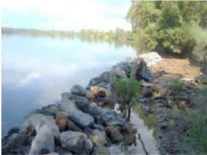
Photo 3-2 Example of rock fillets with timber pins on the Bellinger River in northern NSW
