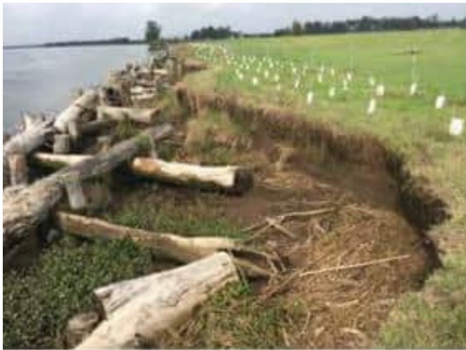
Photo 3-3 Example of log wall on the Hunter River
