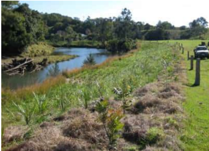
Photo 3-1 Example of bank revegetation and stock management fencing on the Tweed River in northern NSW
