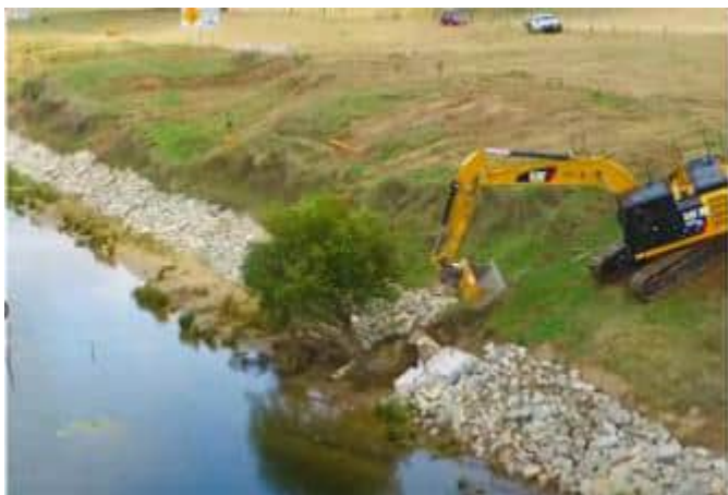
Photo 3-4 Example of lower bank rock toe protection works on the Clarence River in northern NSW
