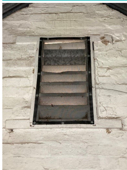
Image 4: Window louvres of the Valve House
