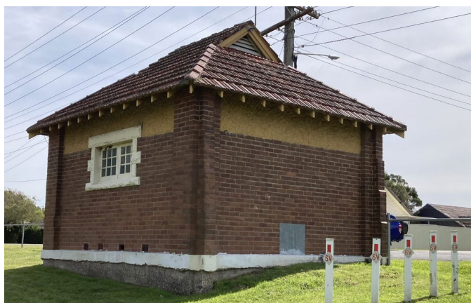
Image 4: View of the rear (southern) elevation showing timber windows with decorative quoins to opening and terracotta vents
