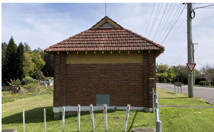
Image 3: View of the eastern elevation of the building showing timber vents
