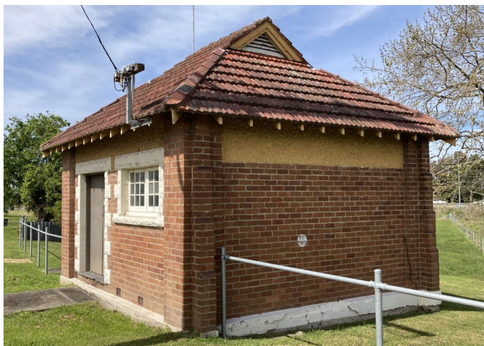
Image 1: View of the northwestern corner of the building showing concrete failure to the western footing
