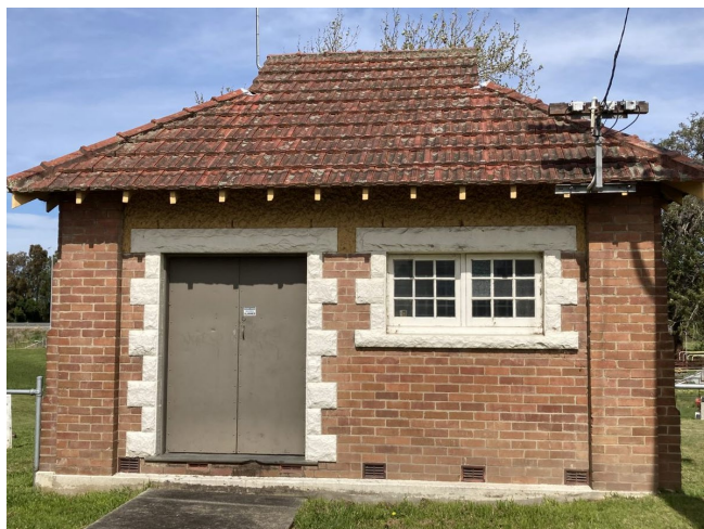
Image 2: View of the principal (northern) elevation showing decorative quoins to openings
