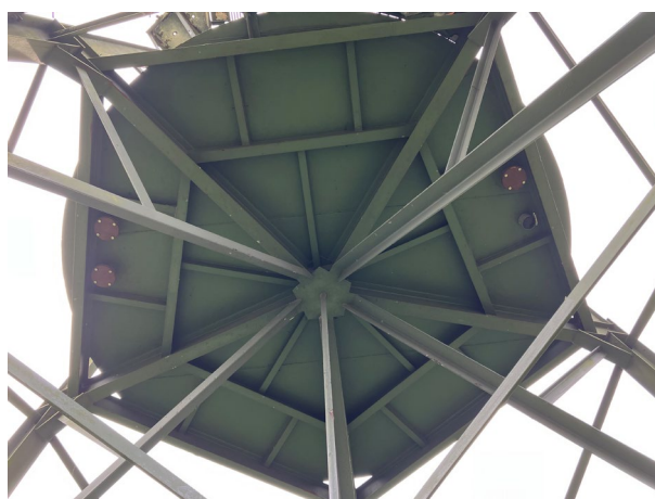
Image 2: Supporting beams beneath the storage tank
