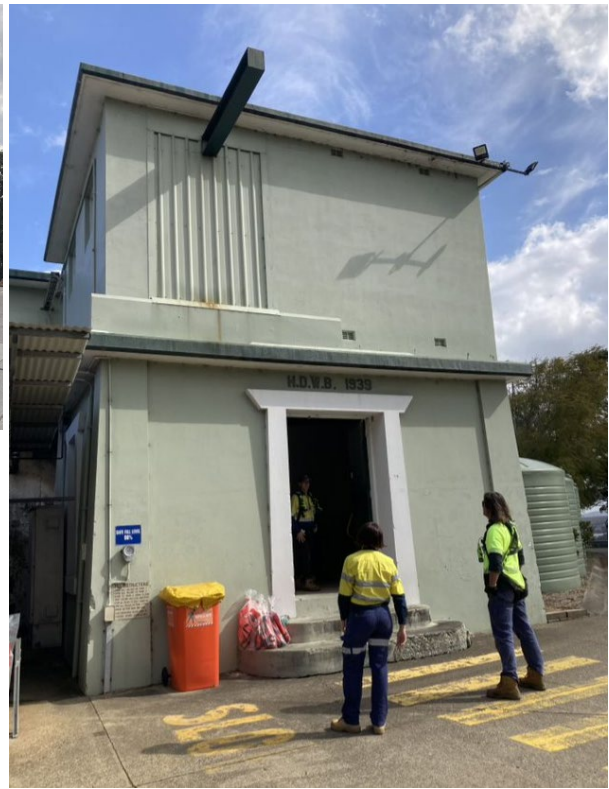
Image 6: Northern elevation of the main valve house showing curved concrete stairs, boarded up opening with gantry and rendered detailing to the entry way
