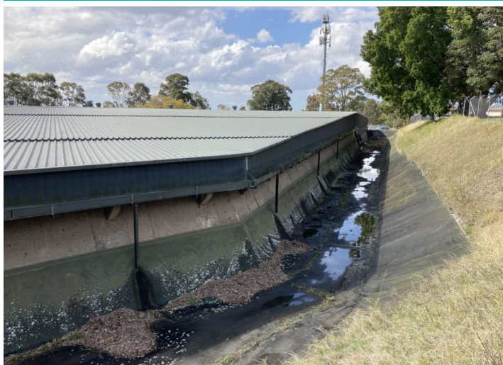
Image 3: View of the southern side of the Reservoir showing the drainage channel lined in geofabric and non-original kliplok roof
