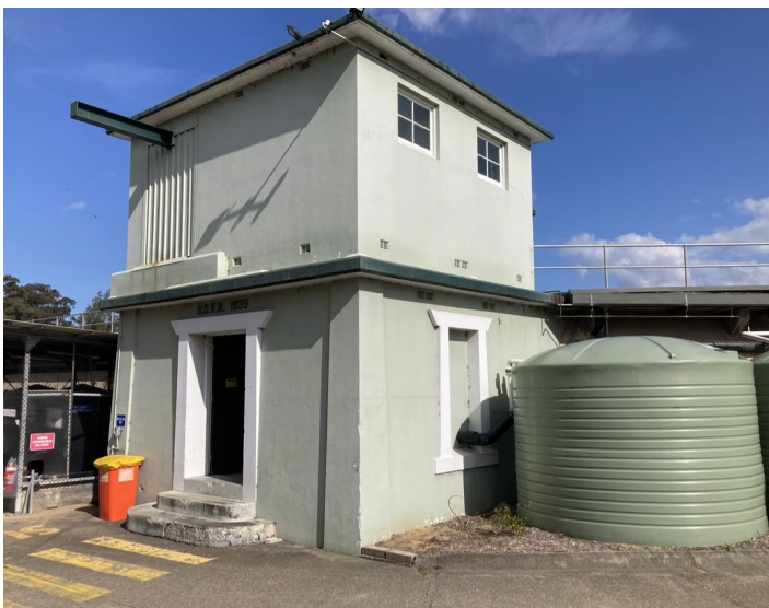
Image 7: View of the main valve house showing architraves, windows, gantry and curved stairs
