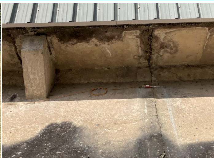
Image 4: Evidence of concrete failure and damage caused by moisture to the soffit and wall of the Reservoir
