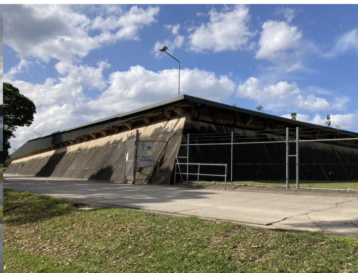
Image 2: View of the southwestern corner of the Reservoir showing the concrete structure with splayed sides
