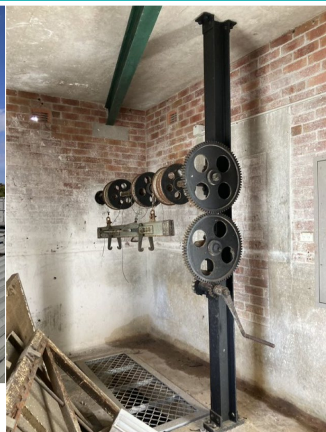
Image 12: Likely original equipment within the annex. Concrete flooring, brickwork walls and concrete ceiling also visible
