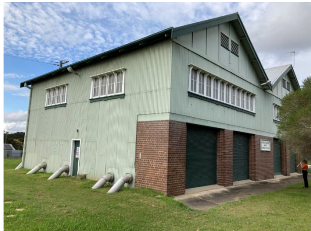
Image 2: Interface between brick detailing and corrugated iron sheets
