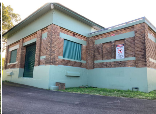
Image 2: Southern elevation of the building (left of frame) and transformer bay (right of frame) showing bricked up and covered windows, roller door, plinth, terracotta vent and recent lighting
