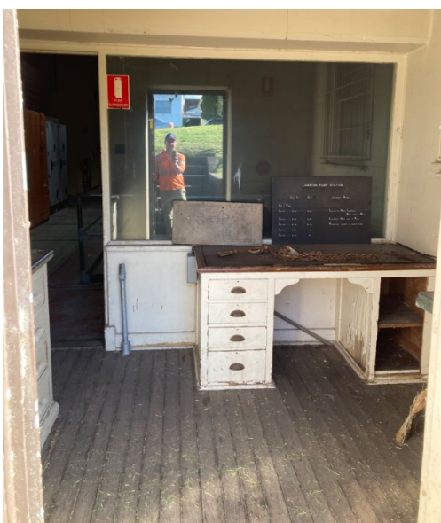
Image 7: Internal view within portico showing timber flooring, furniture and partitions of plasterboard and glazing
