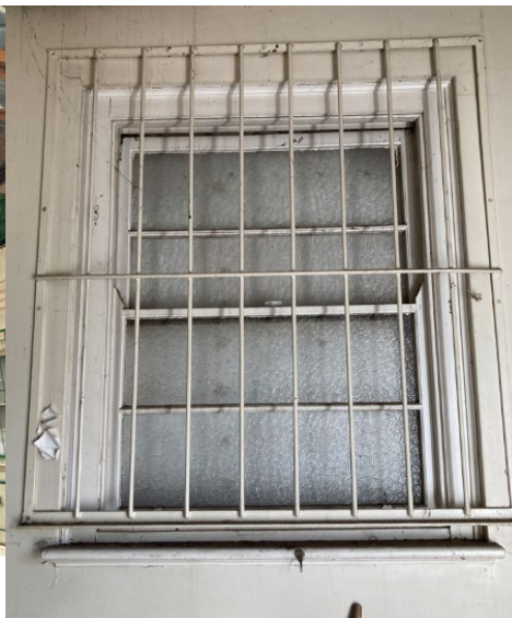
Image 6: Detail view of original double-hung window with timber joinery
