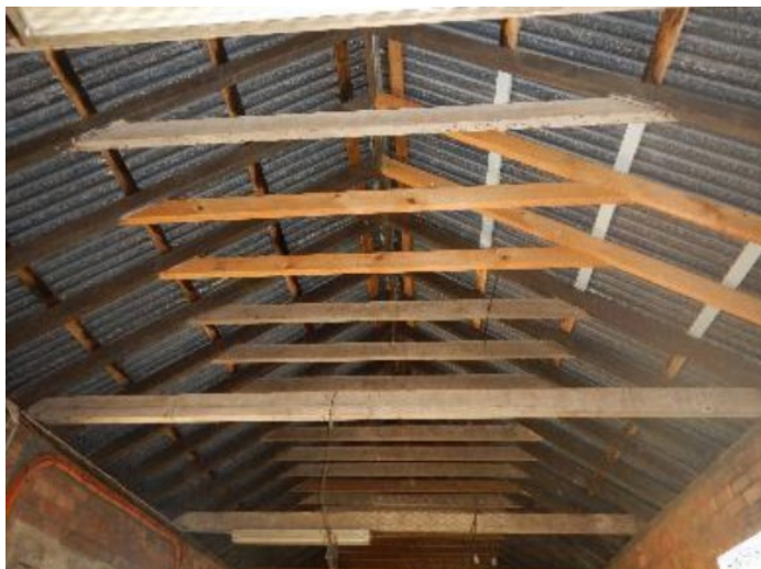
Image 3: Timber roof structure within the northern valve house
