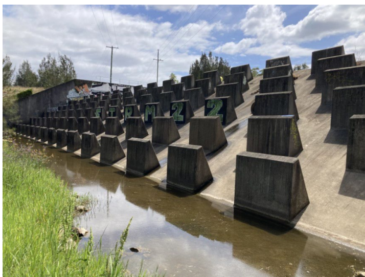
Image 5: Pacific Highway energy dissipator
