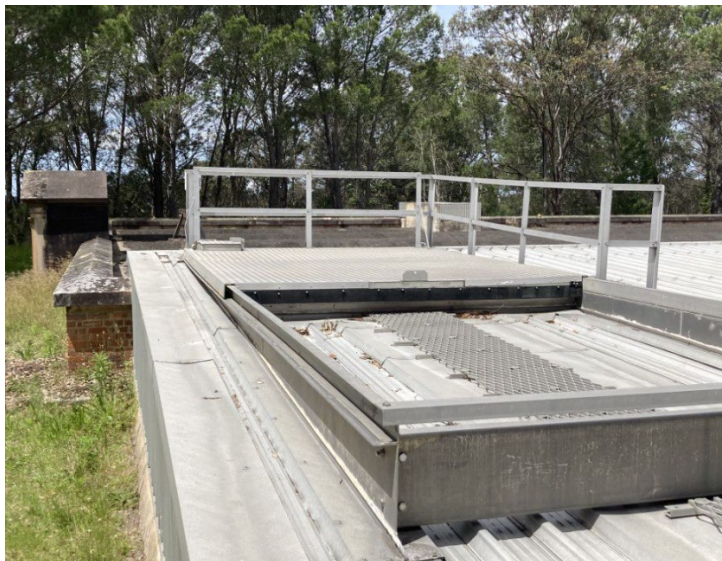
Image 1: Access hatch to roof of Reservoir
