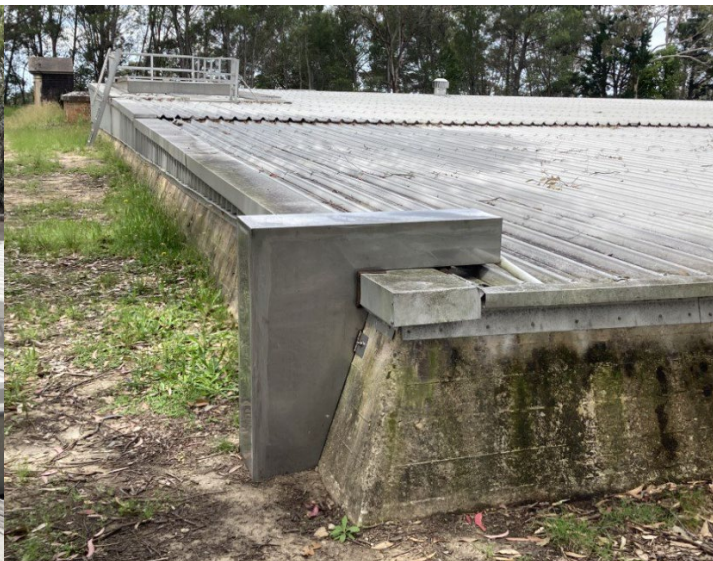
Image 2: Concrete form and later kliplok roof
