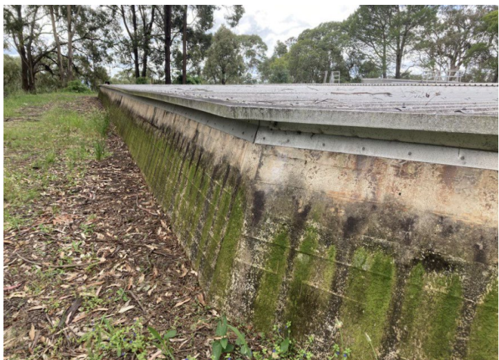
Image 3: Concrete form and later kliplok roof
