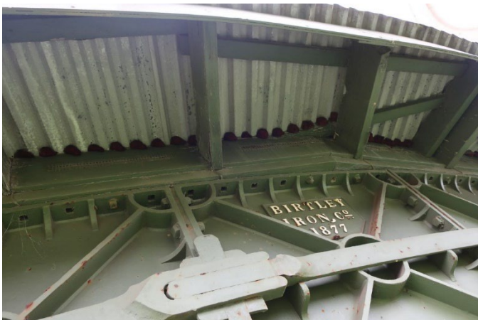
Image 7: Dudley 1 Reservoir contemporary eave detail and maker's mark
