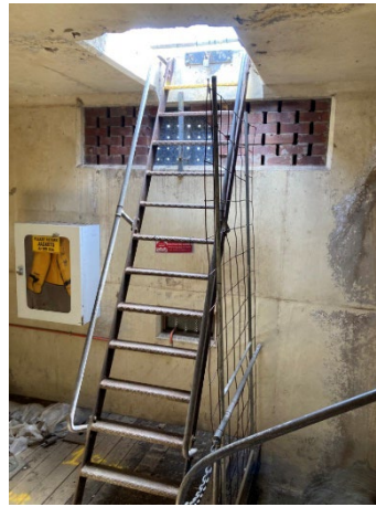
Image 6: Ladder and roof hatch to second storey
