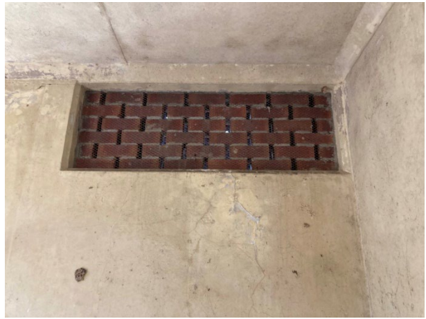
Image 4: Brick infill in window space
