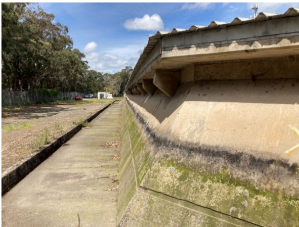
Image 11: Original exposed concrete fascia with 'rafter ends'
