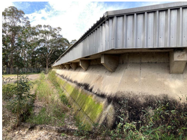
Image 12: Later kilplok roof and fascia
