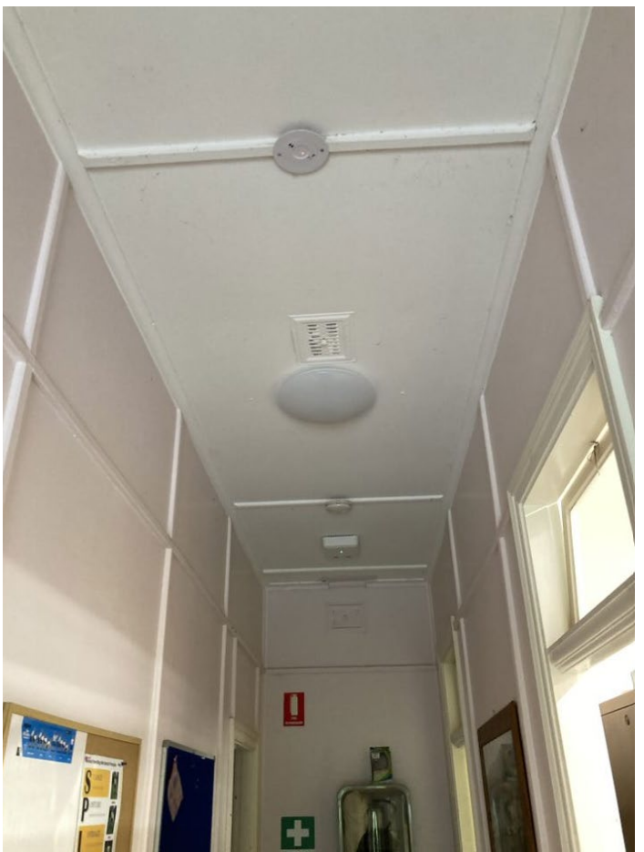
Image 8: Original joinery and ceiling and wall vents to hallway
