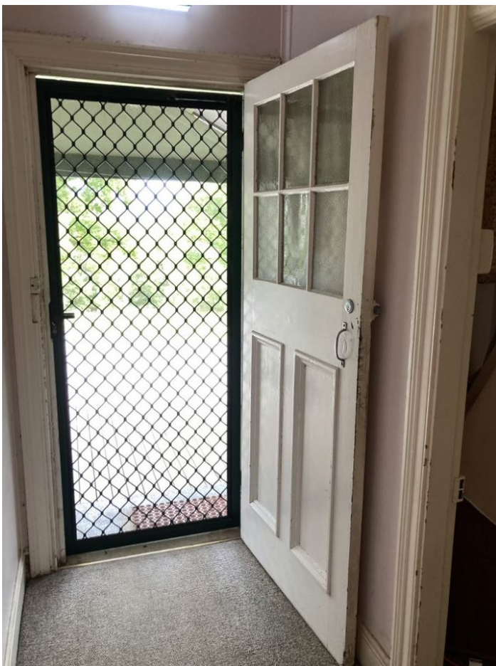
Image 7: Internal original joinery (door, architrave, skirting)
