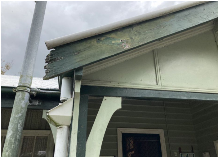
Image 5: Deteriorating timber and timber detailing to portico
