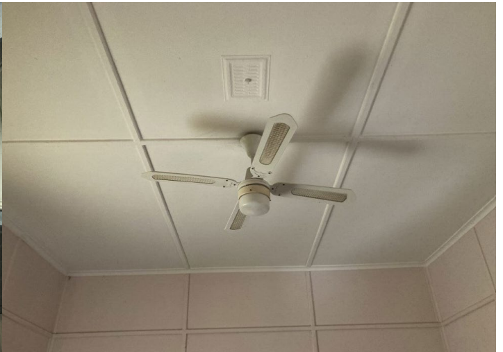
Image 6: Timber batten detailing and vent to ceiling
