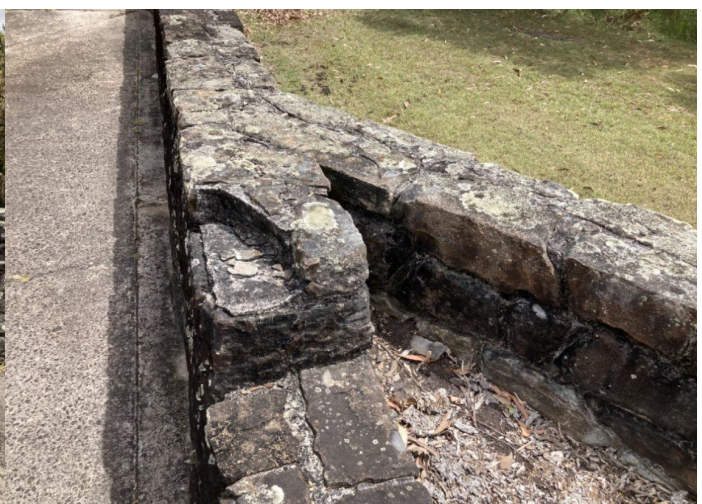
Image 8: Detail view of stone wall showing missing stone
