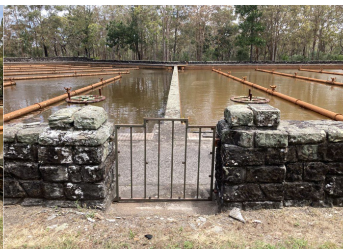
Image 2: View across the basin showing valves, pipes, the weir and the stone wall
