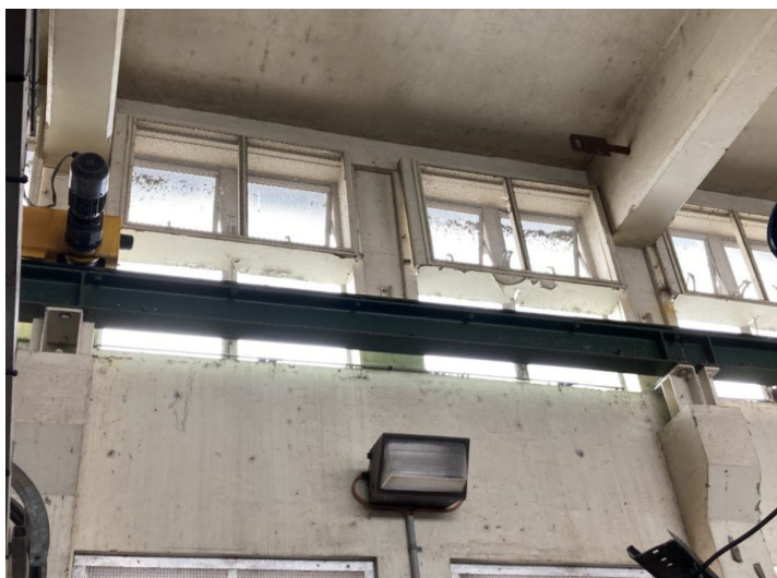
Image 5: Internal view of the side façade showing piers supporting the gantry and multiple rows of windows
