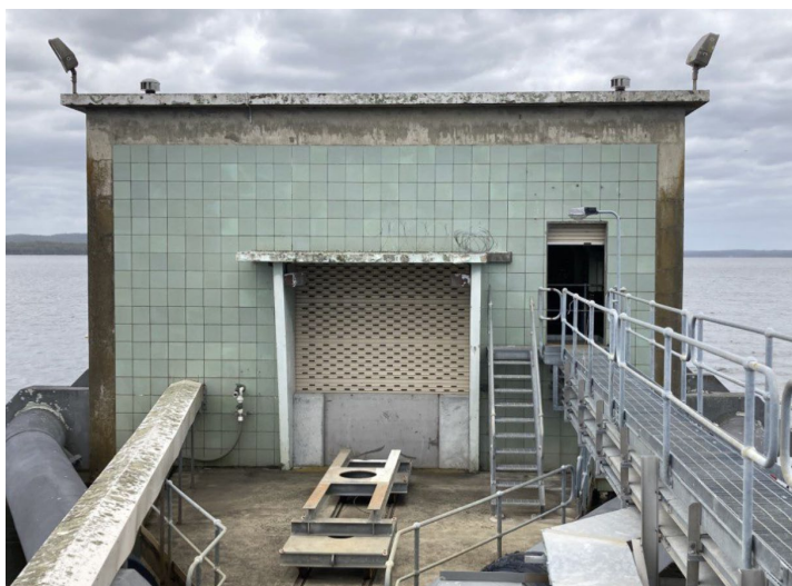
Image 3: Principal façade of the building showing tiles and supported lintel over roller door
