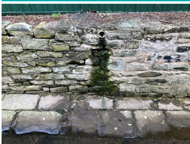
Image 3: Stormwater runoff drain from adjacent property
