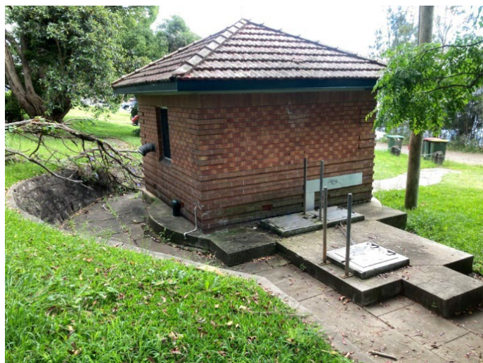
Image 2: Angled concrete footings to accommodate subsurface services
