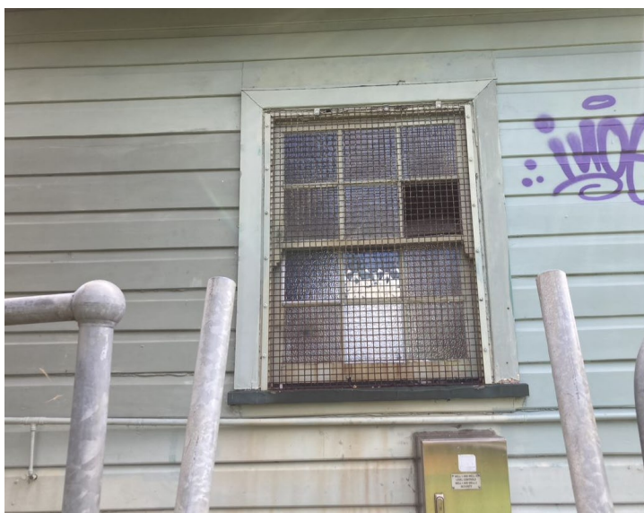
Image 4: View of an original window with later wire mesh added and graffiti to wall
