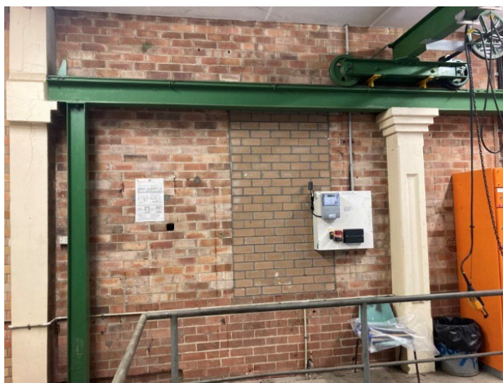
Image 6: Brick infill in window space
