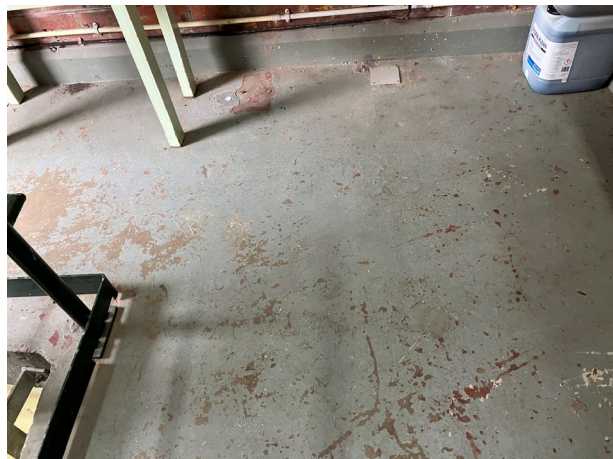
Image 6: Eroding sealant layer on floor
