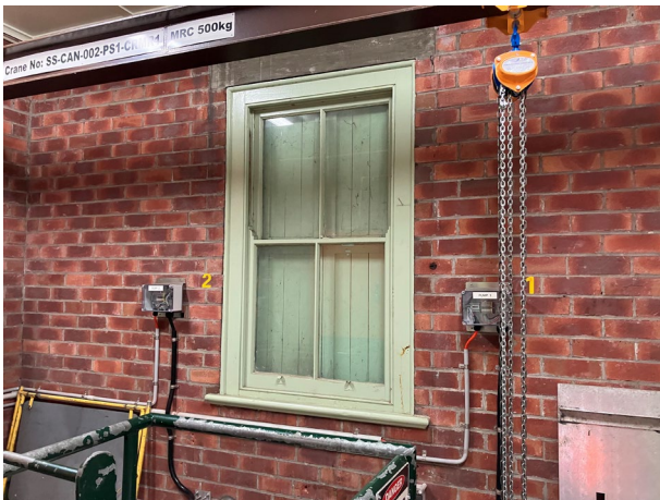
Image 5: Timber sash window
