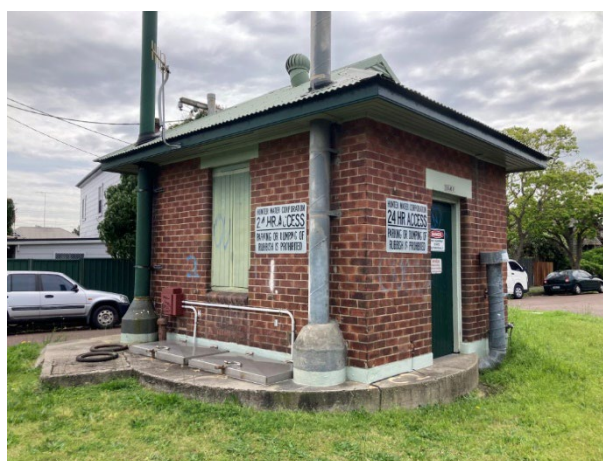
Image 2: Angled concrete footings to accommodation subsurface services
