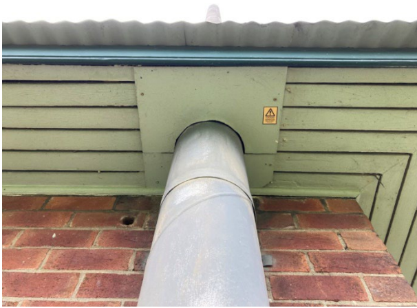
Image 3: Timber panel soffit
