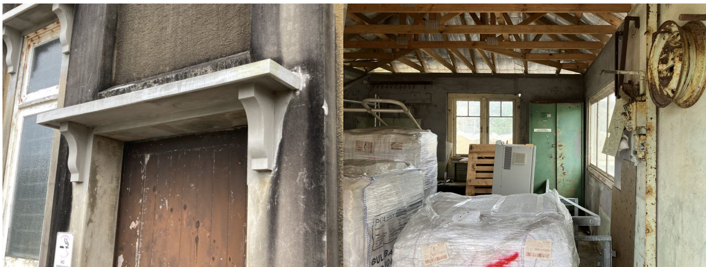
Image 7: Detail of joinery and other decorative elements to the exterior of the Pump House (noting the decorative projecting hood has been sympathetically replaced)
