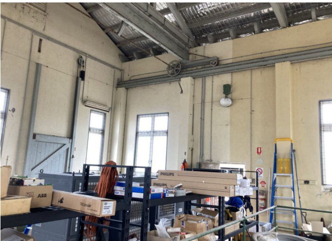
Image 5: Internal view of the Pump House showing gantries, pulley, timber door, original windows and original light fittings
