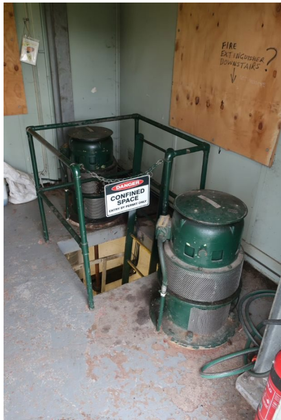
Image 4: Aberdare 1 Waste Water Pumping Station, original ball and pipe handrail around the access to the pit
