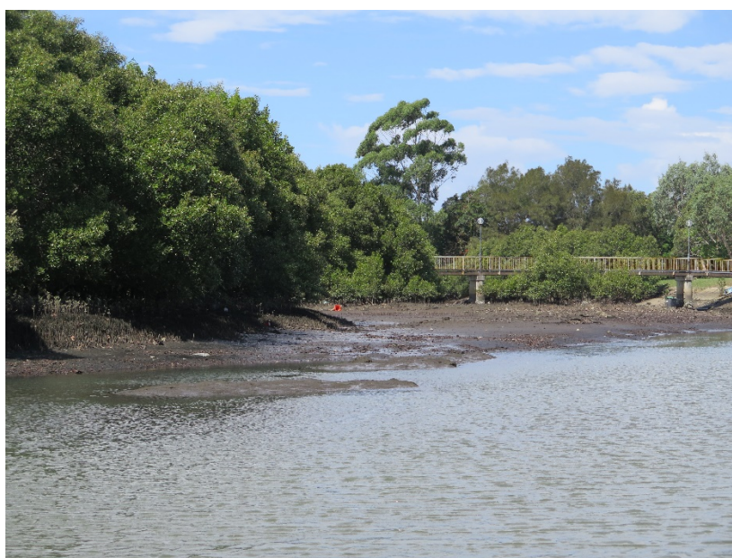
Figure 5-1 Sediment accumulation surrounding Union Street Footbridge
