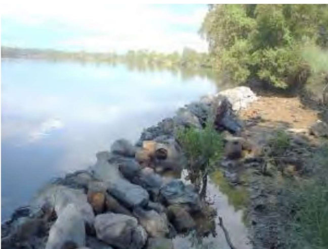
Image 5 - Example of rock fillets with timber pins on the Bellinger River in northern NSW
