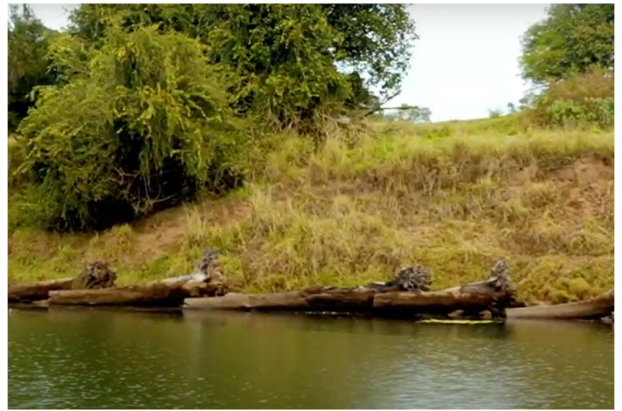
Image 4 - Example of bank toe protection using logs on the Clarence River in northern NSW
