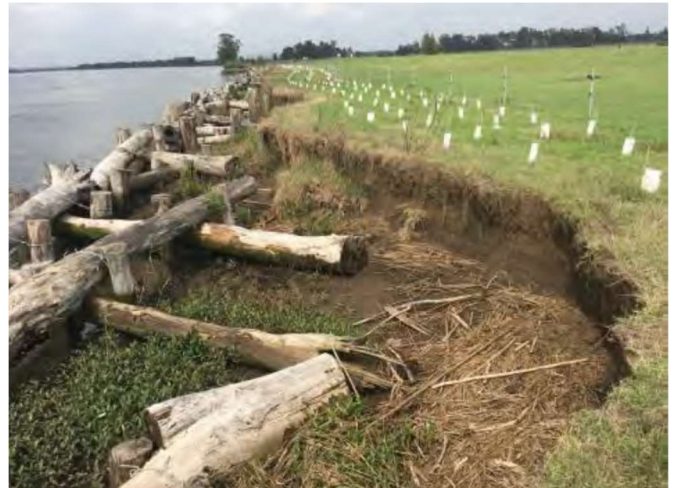
Image 2 - Example of log wall on the Hunter River
