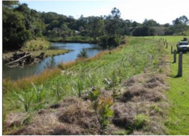
Image 1 Example of bank revegetation and stock exclusion fencing on the Tweed River in northern NSW
