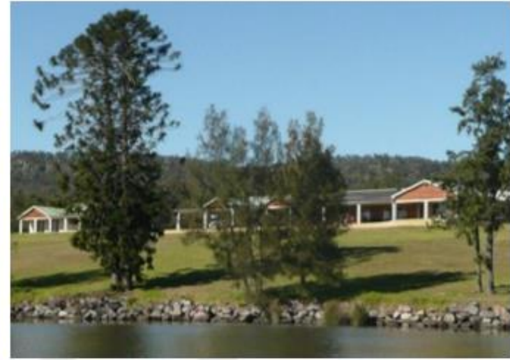
Image 2 Example of established rock revetment on the Williams River
