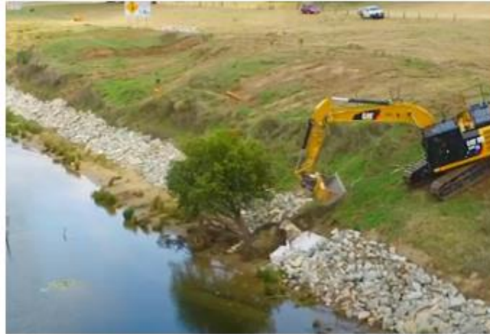
Image 3 Example of lower bank rock toe protection works on the Clarence River in northern NSW
