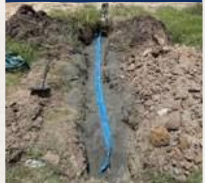
Open trench: marking tape
