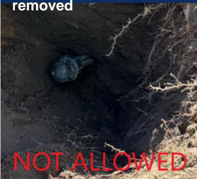
Not Allowed – Dead legs, they must be removed
