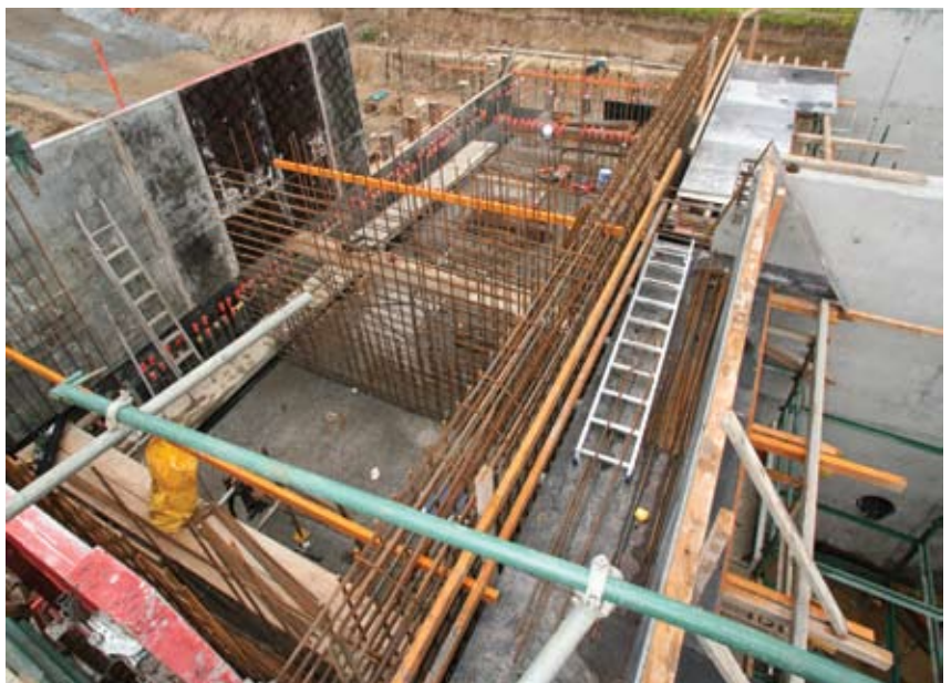
> Works in progress at Branxton wastewater treatment works
