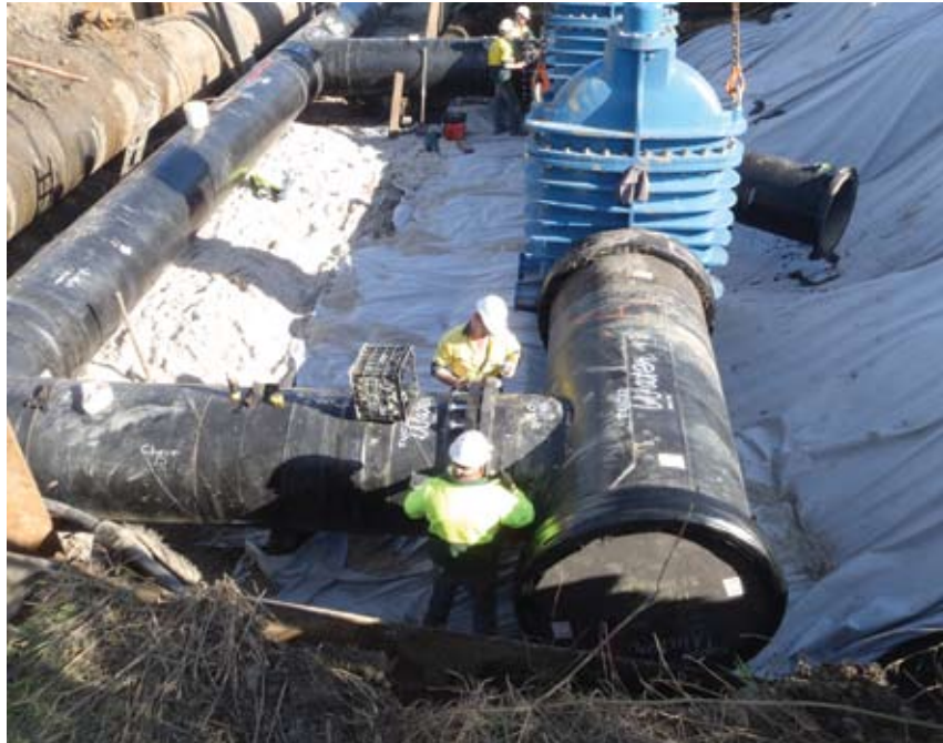
> Installing the new 900mm watermain into the existing system at Shortland
