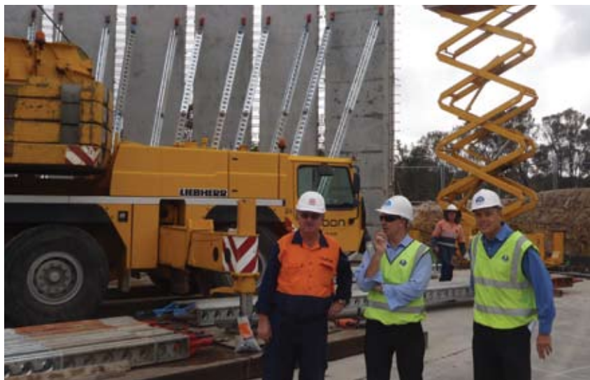
> Anna Bay reservoir works in progress
