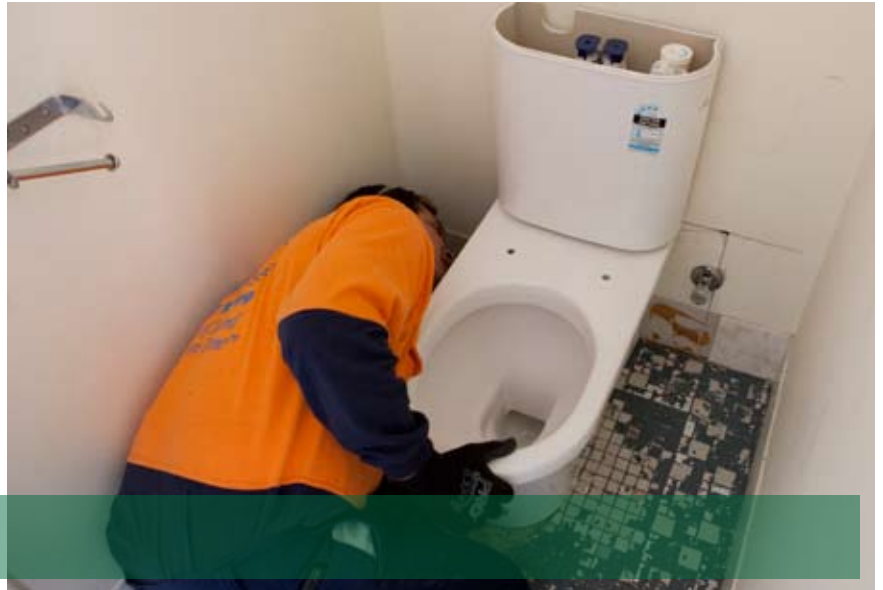
REPLACING THE OLD TOILET
