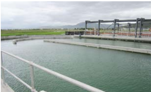
Mt St John Wastewater Purification Plant won the Engineers Australia Townsville Regional Project of the Year Award 2012.
