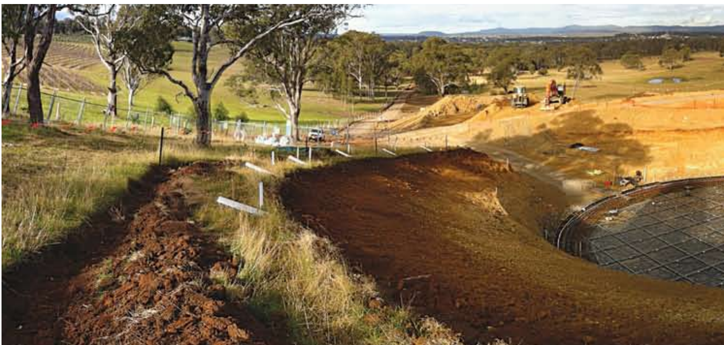
Cessnock Reservoir works in progress.
