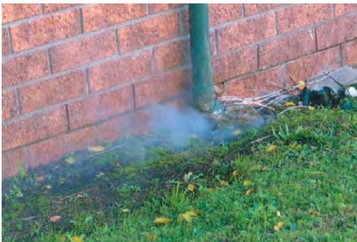
*Smoke can reveal faults that allow stormwater into the sewer system*
