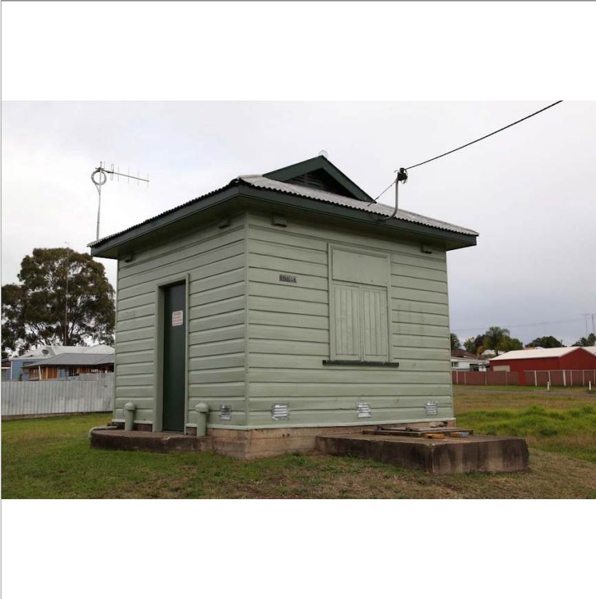
Cessnock 2 Waste Water Pumping Station
