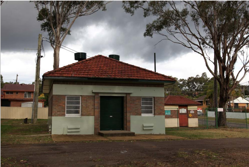
Bellbird Water Pump Station
