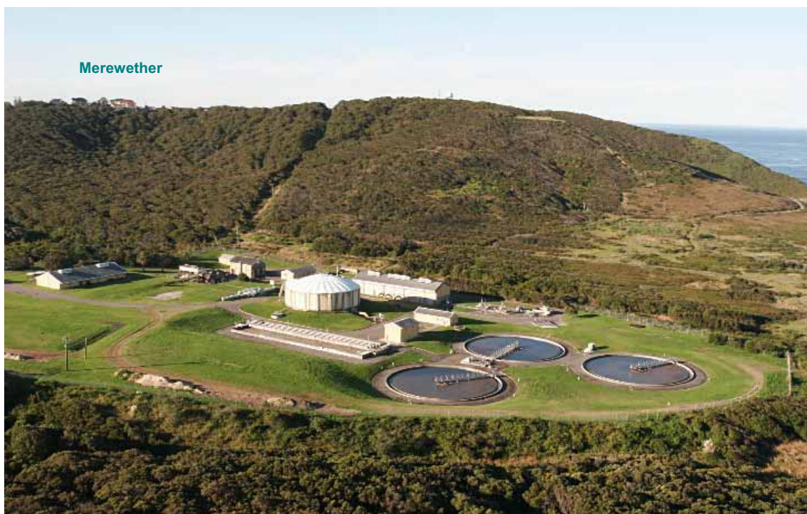
Figure 1-2 Aerial View of Existing Burwood Beach WWTW
